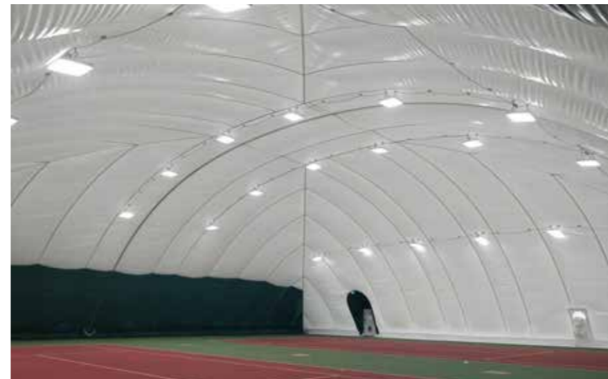
INTERNAL OF TYPICAL AIRDOME
