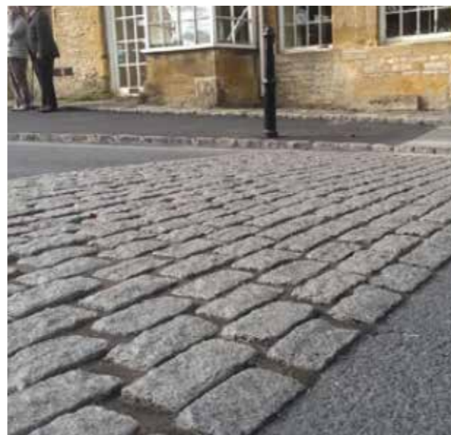
Granite setts to traffic calming area
